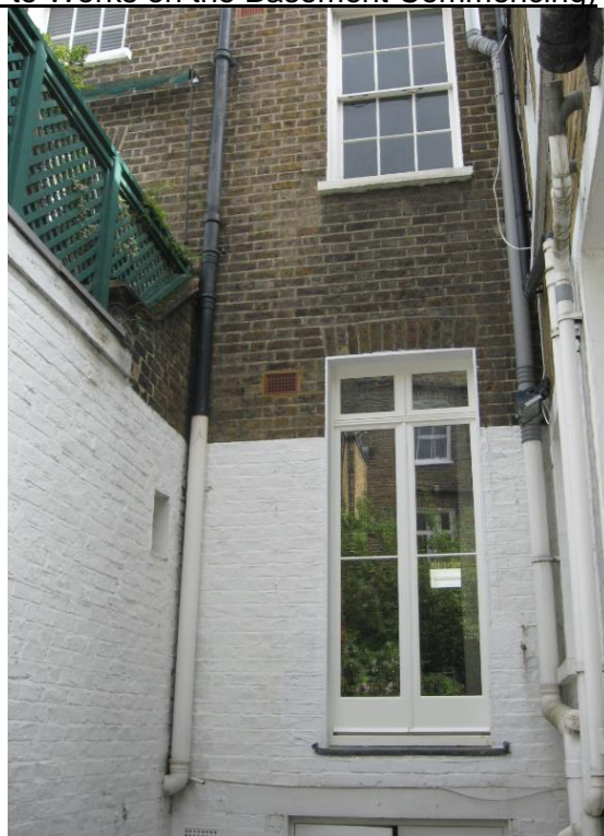
Rear Elevation (Prior to Works on the Basement Commencing)
